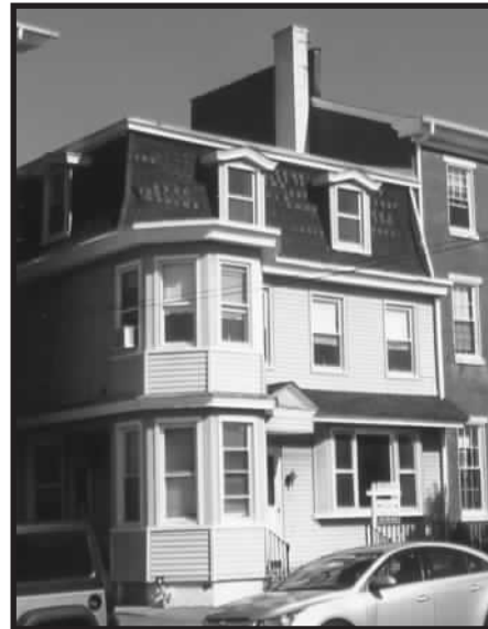
House in the 400 block of Radcliffe Street
