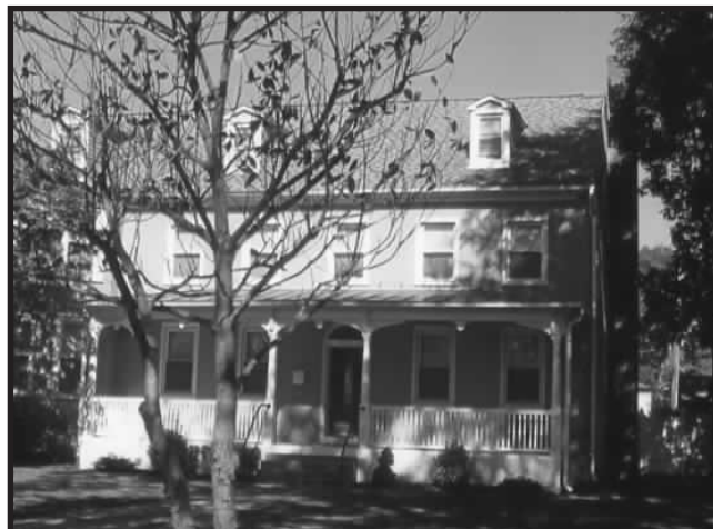
House in the 900 block of Radcliffe Street
