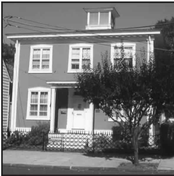
House in the 300 block of Radcliffe Street
